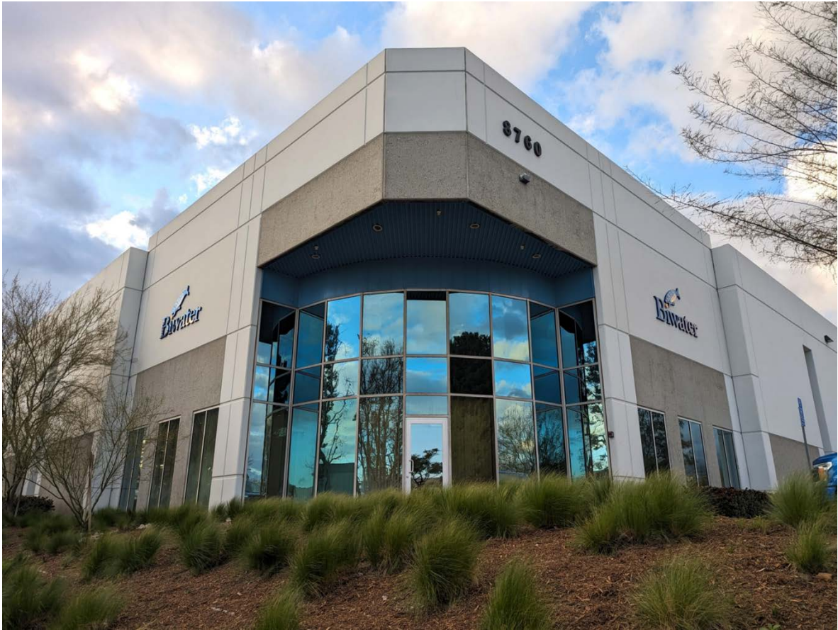
Caption: Biwater Inc's. new facility in Rancho Cucamonga, California
